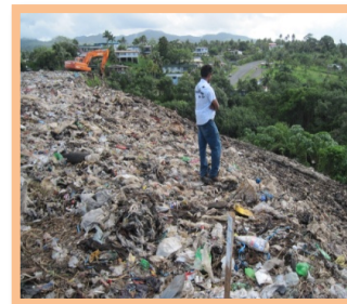
Lami Rehabilitation work.
