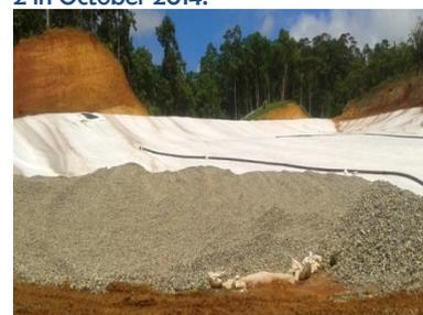
Figure 26.0: Preparation of the landfill for filling
